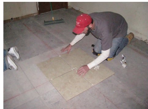
A new ceramic tile floor is installed during kitchen renovation.
